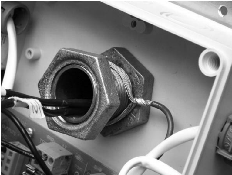
Figure 8: Mounting Sequence, Inside Rear of Fuse Box
