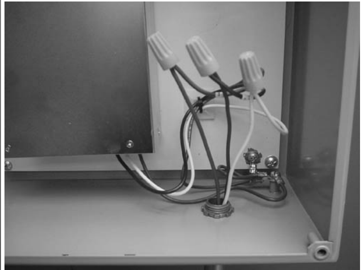
Figure 2: Grounding Post Locations
