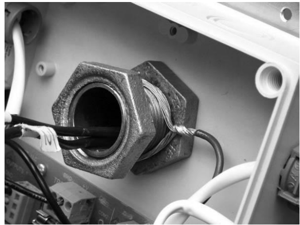
Figure 9: Mounting Sequence, Inside Rear of Fuse Box
