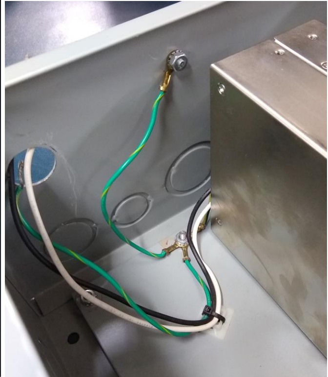
Figure 5: Grounding Post Locations
