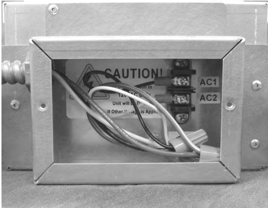
Figure 9: Completed Wiring in Junction Box
