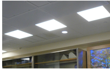
FIXTURE TYPE High-Bright Troffers
