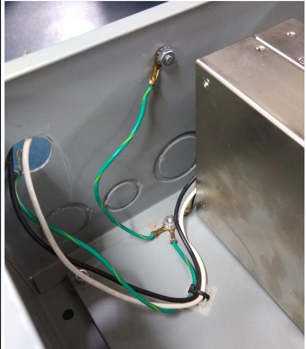
Figure 5: Grounding Post Locations
